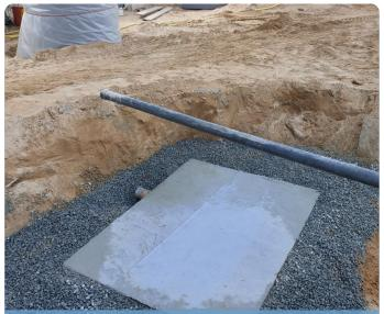
Gravel aggregate to protect the tank from blockages
