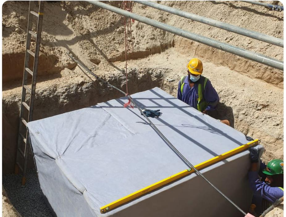
Polystorm geocellular tank - a SuDS solution
