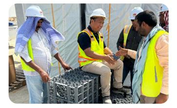
What's more, we were even able to reduce the cost of this more advanced solution through value engineering. In order to ensure that the Polystorm geocell could withstand heavy load capacities, the tank had to be installed deep underground. As a result, it was originally thought that PSM5 would be required, however our technical team assured them that PSM1, with its 40 tonnes/m<sup>2</sup> compressive strength, was more than adequate for the application.
