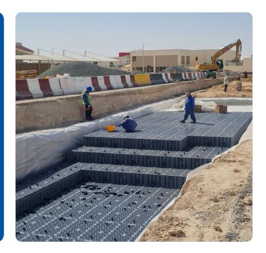
Given the RTA's sustainability focus, Polypipe Middle East emerged as the ideal partner to implement a comprehensive stormwater management system. This system goes beyond mere flood prevention and includes the installation of multiple stormwater tanks at four locations along the AI Lesaili community's internal roads during construction. This is phase one of an internal roads project that additionally includes Margham, Lehbab, Nazwa, and Hatta.
