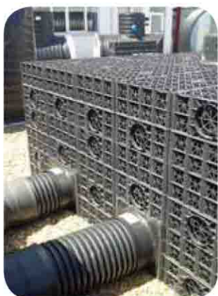
Typical Polystorm 450mm inlet manifold detail
