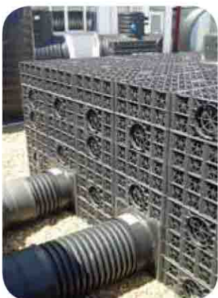
Typical Polystorm 450mm inlet manifold detail
