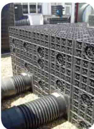
Typical Polystorm 450mm inlet manifold detail
