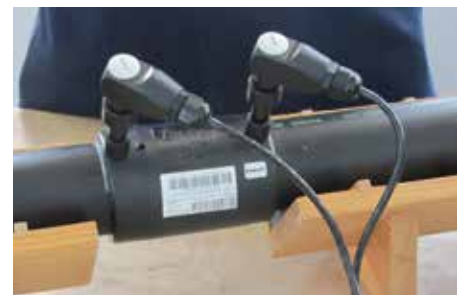
Finished electro fusion weld
