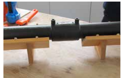
Electro weld process
