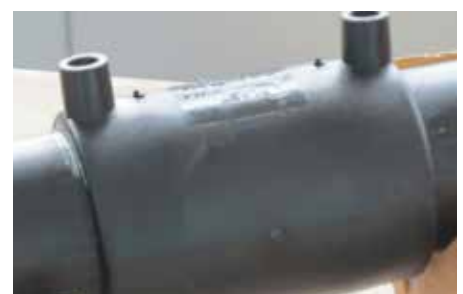
Finished electro fusion weld
