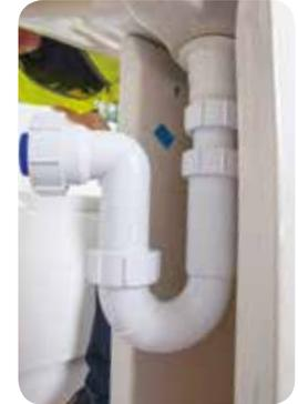
4. To connect your trap to your waste pipe remove the threaded nut on the outlet of the trap, along with the blue finned rubber seal, and blue spacer. Place the threaded nut over your waste pipe, with the exposed threads
