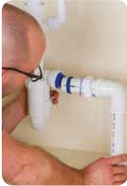
nut has been hand tightened a final ¼ turn is required. A final inspection of the connection is required to make sure the connection has been made by pulling on the pipe and fitting. This may not be suitable in certain applications.
