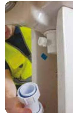
2. To complete the installation, thread the nut onto the outlet. There should be no play in the connection between the outlet and the trap.
