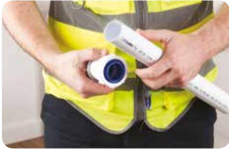
2. Remove threaded nut, washer and seal from the fitting.
