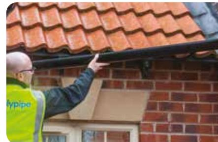
4. Once the back edge of the gutter is in place, the front edge can be clicked into place. It's best to have your gutter in the correct position prior to connecting the front edge as it can be difficult to move the gutter along the run of fascia brackets once it's in place.
