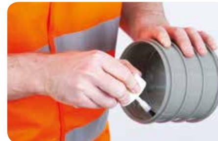
4. Apply a coat of Polypipe solvent cement to both surfaces to be jointed using the brush applicator provided in the lid. The cement should be applied along the length of the spigot and not around its diameter.
