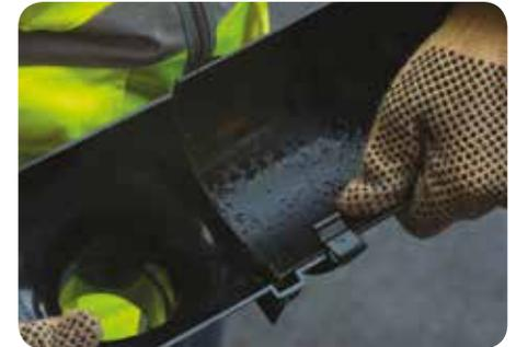
5. It is also important that the gutter is not connected beyond the expansion line which is clearly marked on each fitting.
