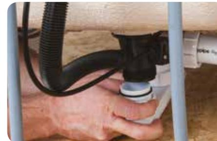
8. To complete the installation, thread the nut onto the outlet. There should be no play in the connection between the outlet and the trap.
