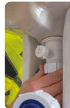
3. If you have installed an adjustable trap as we have in this installation then the trap can be positioned in line with the waste pipe. To do this, loosen the threaded nut below the threaded nut that is connected to the outlet. Then move your trap either up or down as required, once this is complete re-tighten the threaded nut to re-seal the trap.
