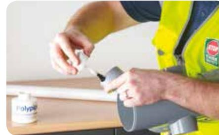
6. Insert the boss adaptor into the boss socket on the soil fitting. Remove any excess solvent cement.
