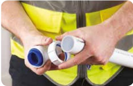
3. Place the threaded nut first onto the pipe, then the blue washer. Finally push the seal onto the pipe with the seal facing into the fitting.
