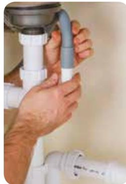
7. When connecting your trap to your waste pipe it's important that the pipe can be fully inserted into the outlet of the trap. Once this has been done you can then move the blue finned seal along the waste pipe into the trap. Once the seal is in place, the threaded nut can be threaded onto the trap, which will create a compression seal between your waste pipe and trap. After the threaded
