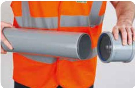
3. Lubricate the spigot or ring seal with Polypipe silicone grease or aerosol lubricant.
