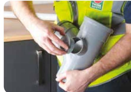
7. Once the boss adaptor is inserted into the boss socket on the soil fitting, ¼ turn the boss adaptor. This process is important as it helps achieve a tighter bond between the boss connector and the soil fitting.
