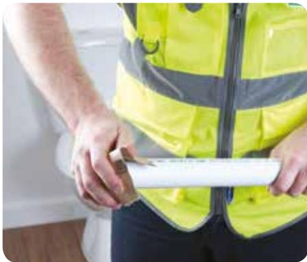
3. Lubricate the spigot or ring seal with Polypipe silicone grease or aerosol lubricant.
