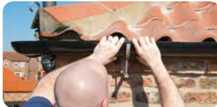
Standard rafter brackets only fit around gutter, not fittings. It is necessary to use the universal rafter brackets to connect unions and running outlets.
