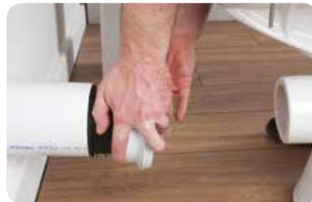
3. Once the pan connector is inserted into the pipe the toilet can be positioned and installed to the pan connector.
