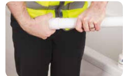
6. Any surplus solvent cement should be removed with a clean synthetic cloth.
