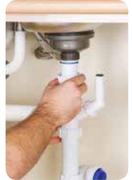
4. Fully tighten your threaded nuts. There should be no lateral movement between these parts once they are installed correctly.
