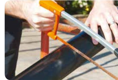
2. After your gutter has been cut we recommend removing any burrs that may be present with a piece of sandpaper. This will stop any loose bits of plastic cutting into the seal.
