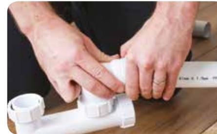
6. A final inspection of the connection is required to make sure the connection has been made by pulling on the pipe and fitting. This may not be suitable in certain applications.
