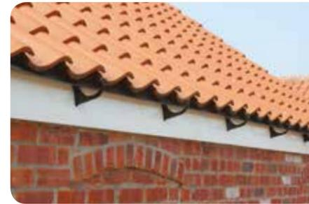
All supports should be fixed at centres not exceeding those detailed in table 11 opposite as well as adjacent to both ends of any gutter angles.
