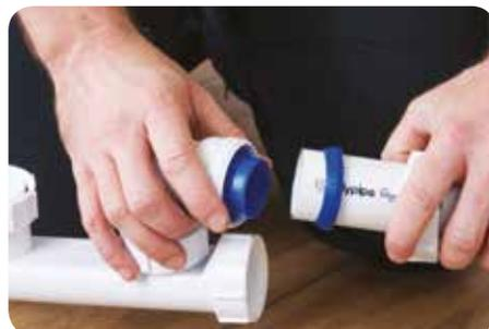
5. Once the seal is in place, the threaded nut can be threaded onto the trap, which will create a compression seal between your waste pipe and trap. After the threaded nut has been hand tightened a final ¼ turn is required.
