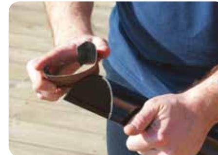
3. Polypipe rainwater systems are fitted with a flexible clip and seal jointing mechanism, making it easy to connect gutter to fittings. Because the clip is flexible and not part of the body of the fitting this allows for much easier installation.
