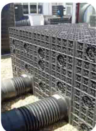
Typical Polystorm 450mm inlet manifold detail
