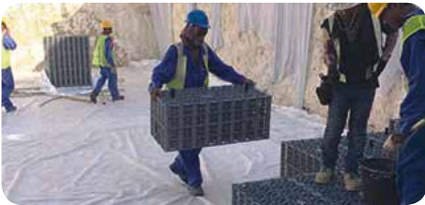
3 Install light in weight units one at a time
