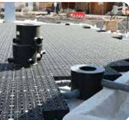
Permavoid installation
