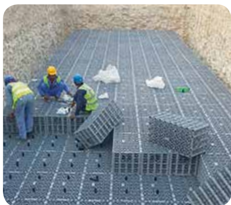
Polystorm installation
