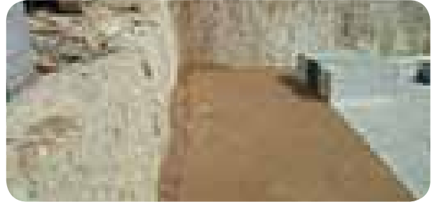
2 Excavation, base preparation and geotextile fabric
