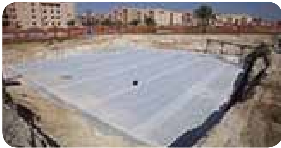
9 300 GSM geotextile should encapsulate tank (minimum 300mm overlap)
