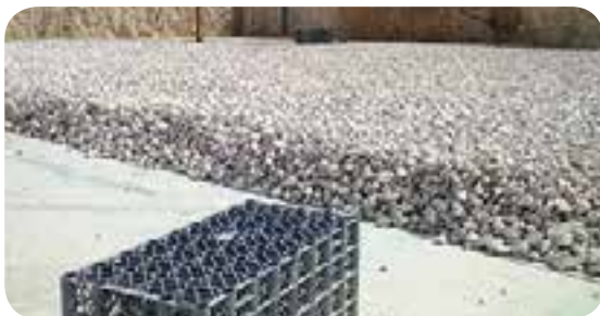
13 Continue backfilling on top of completed tank (refer to design for minimum depth)
