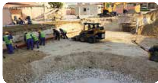
14 Continue backfill compaction with clean excavated material
