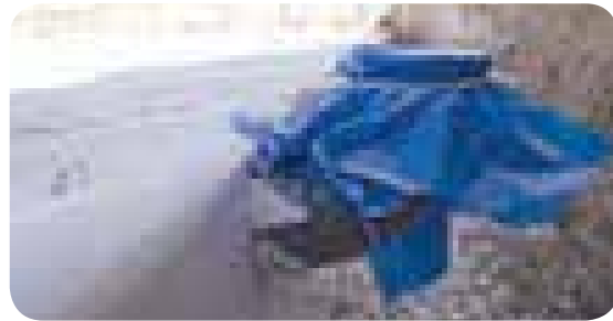
10 Geotextile 'star cut' should be made for pipe connections and vent pipes
